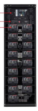
the state of charge (SoC) and state of health (SoH). It also contains a molded-case circuit breaker and a shunt resistor. The SMPS supplies the power for the BMS and communicates with the UPS and other connected cabinets. Battery cabinets may be connected in parallel to achieve the power needed.
