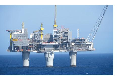
Troll A is a majestic construction, 472 meters high, with an underwater concrete structure to 369 meters depth and a dry weight of 656 000 tons.
