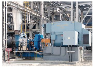
Pump motor soft started by the ACS5000 to reduce mechanical wear and tear.
