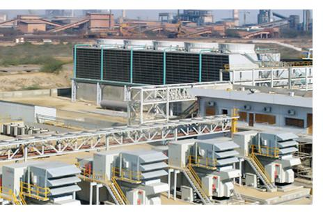
Al-Tuwairqi Steel Mill Ltd suffers from an electricity network that restricts direct-on-line startup of its medium voltage motors. The reliability and availability of an ACS5000 drive system is called upon to provide soft start without increasing operating costs or further impacting on the network.
