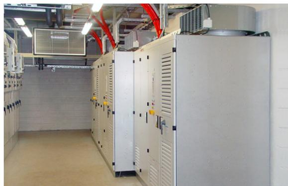
03 Control room with ACS2000 variable speed drives (left) and UniMix switchgear (right).
