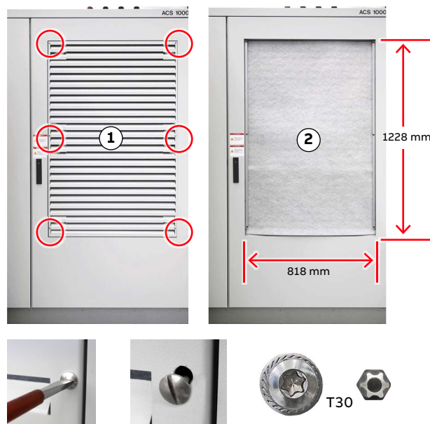
Fig. 74. Filter panel (1) and filter mat (2) on rectifier and inverter compartment
