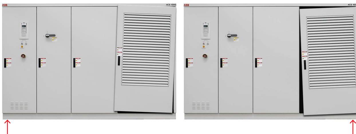
Fig. 40. Leveling the drive
