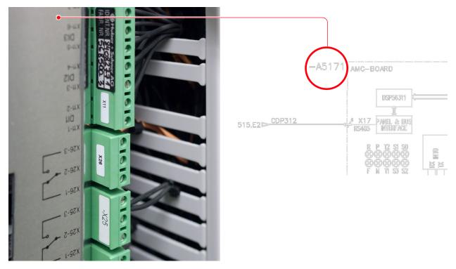
Fig. 72. Device identification
