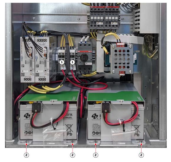
Fig. 78. Control compartment - replacing the batteries
