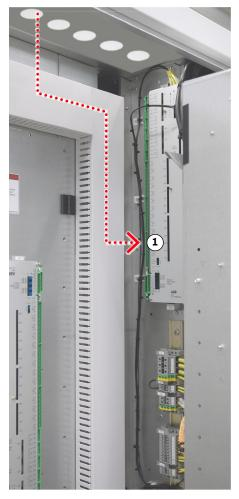
Fig. 60. Cable entry from (A) top, from (B) bottom
