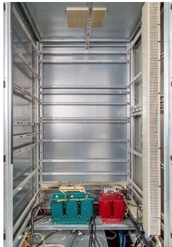
Removal of control electronics
