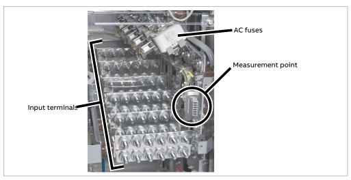
two supply module cubicles, and three measurement points (XAC1, XAC2, XAC3). The picture below shows a cubicle with two modules.
