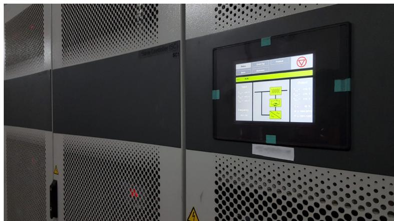
ABB's PCS100 AVC-40 protecting against voltage sags at a leading semiconductor test assembly company in Malaysia
