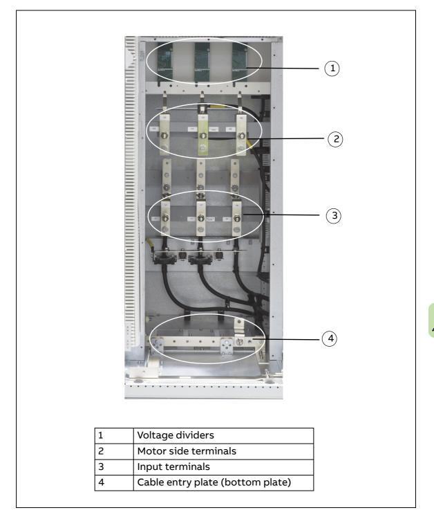
*Terminal compartment with cover plate removed, view from front.*
