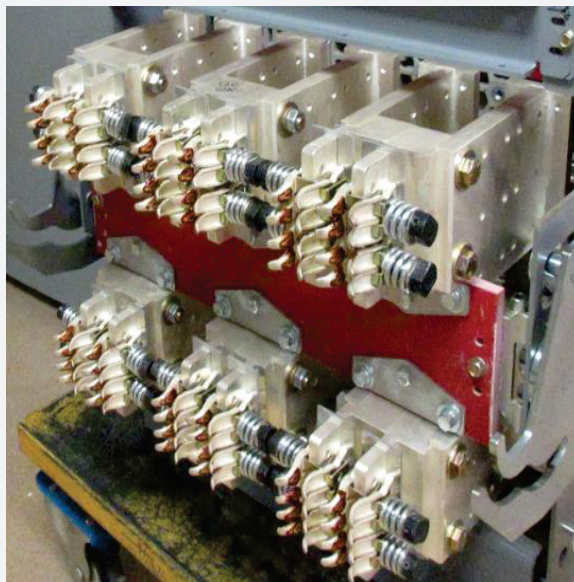
Primary Contacts or “Fingers” (Apply Grease to sliding surfaces)
