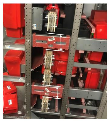
Access for connect the links of Bus Bars
