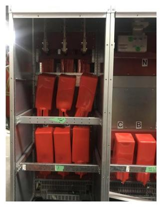
Insulation Boots and Cable Supports to be removed
