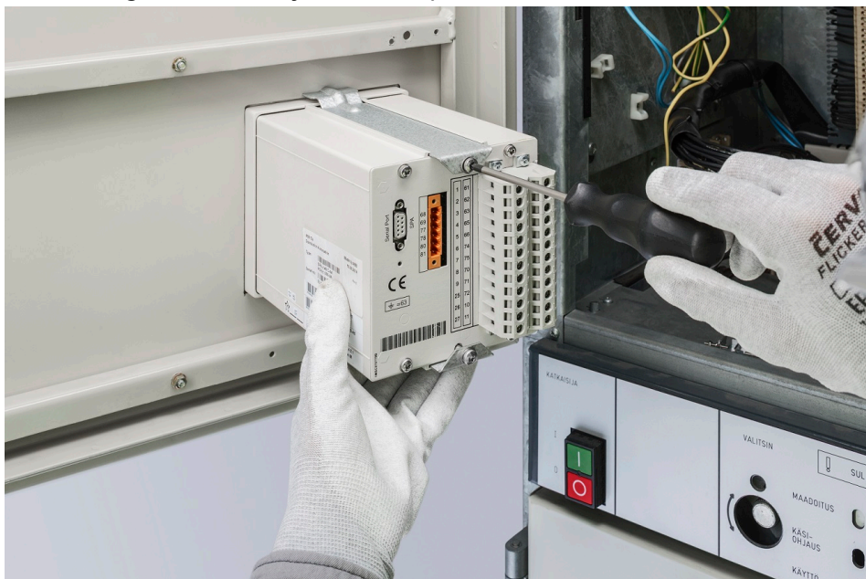
Figure 9: Loosening the fixing screws of SPACOM relay and detaching the fixing parts
