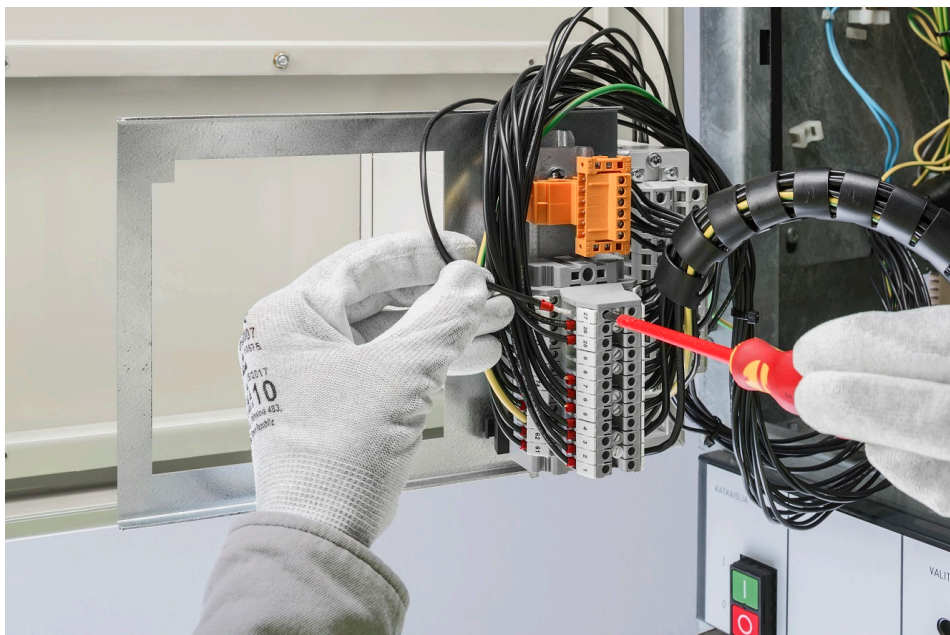
Figure 7: Connecting all wires to the corresponding terminal of the relay retrofit adapter set by following the terminal numbering
