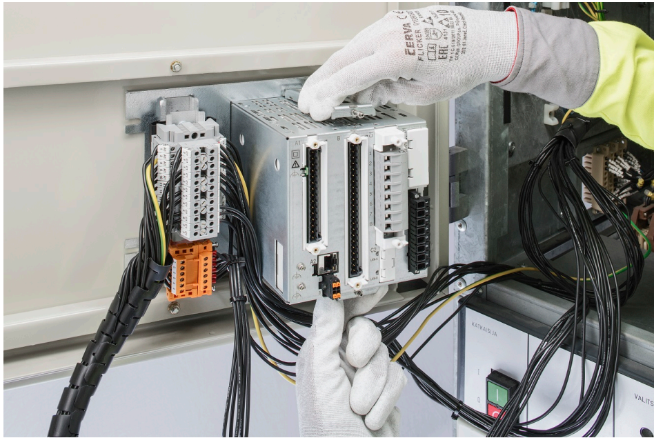
Figure 18: Mounting the fixing clamp assembly together with the relay retrofit adapter set
