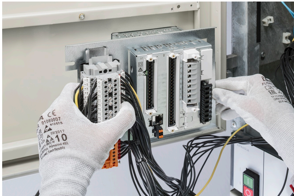
Figure 16: Inserting the relay retrofit adapter set around the REX610 relay (for example purposes only)
