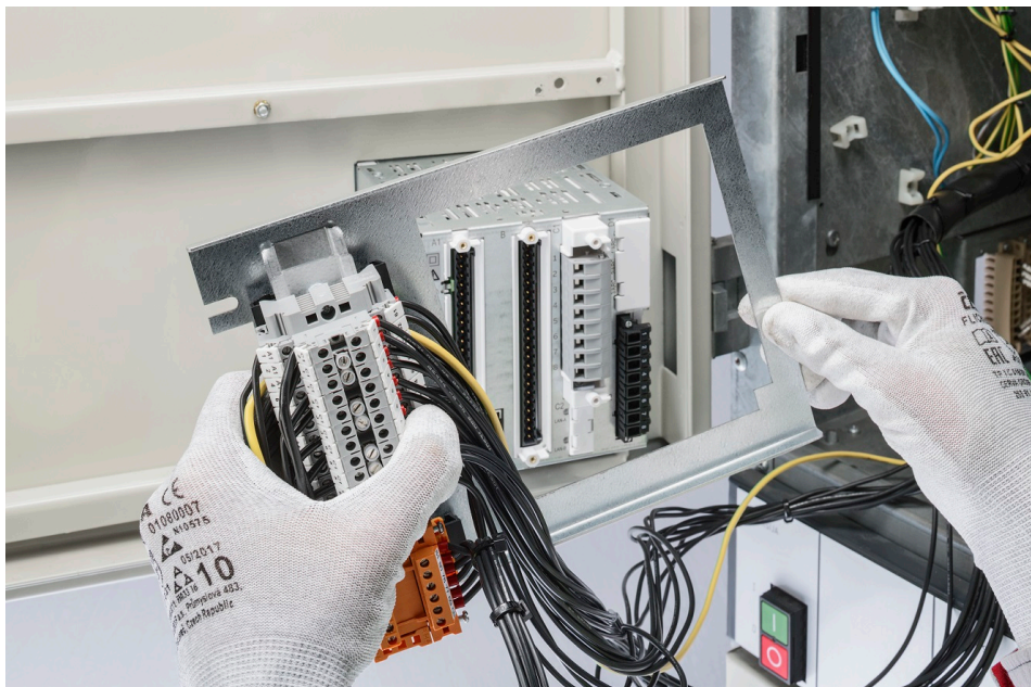
Figure 15: Deciding the correct direction of the relay retrofit adapter set installation
