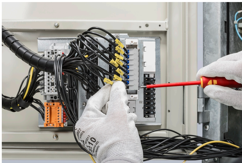
Figure 22: Connecting the pre-wired CT/VT wires to the REX610 CT/VT connector by following the markings
