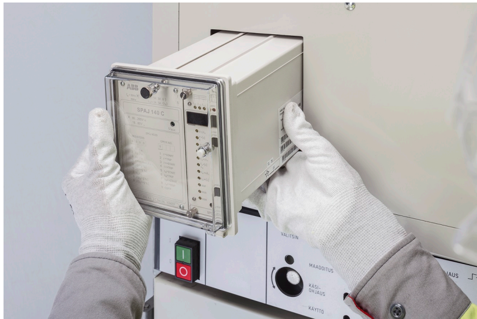
Figure 10: Taking out the SPACOM relay from the existing location
