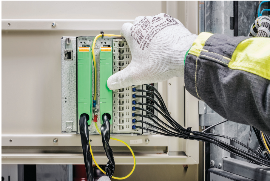
Figure 4: Earth lead connected to the earth screw
