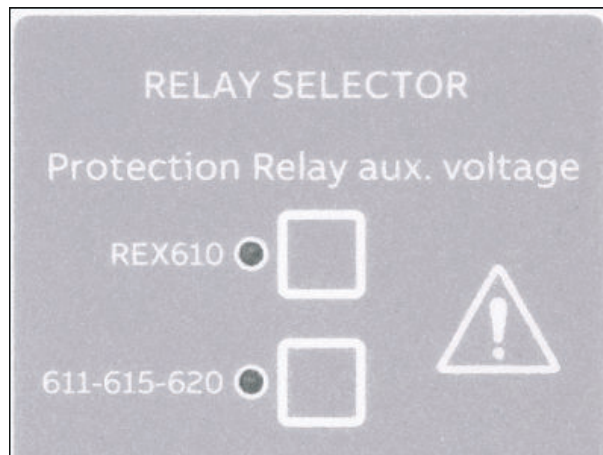
Figure 7: Voltage selector for the relay's auxiliary supply voltage
