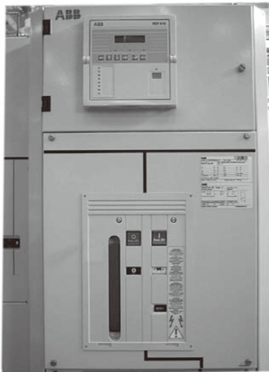
V-module with protection relay type REF610 in integrated LV-compartment with hinged door
