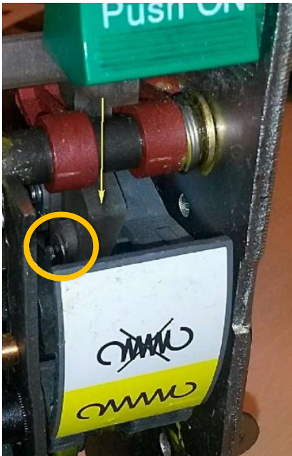
Figure 25 - Anti-reclosing function verification
