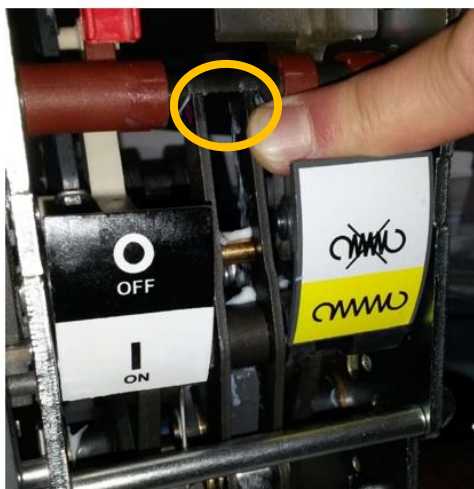
Figure 26 - Opening function verification
