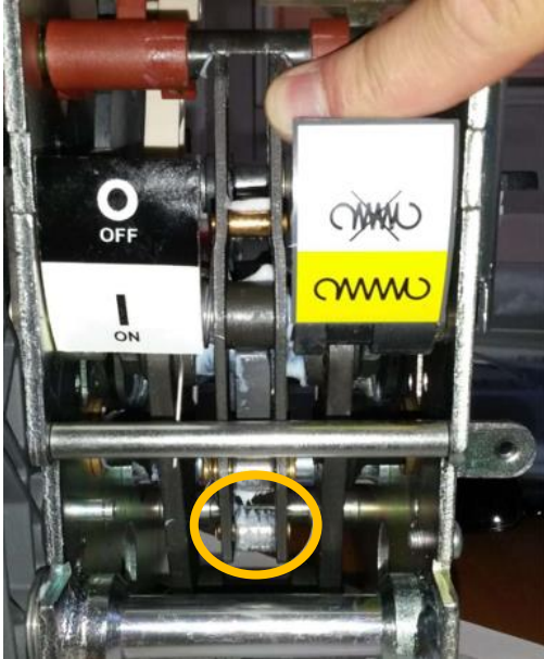
Figure 23 - Rollers cleaning
