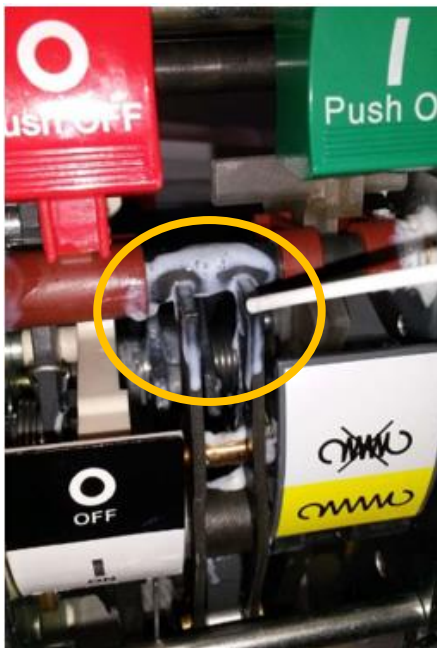
Figure 30 - Hooks greasing
