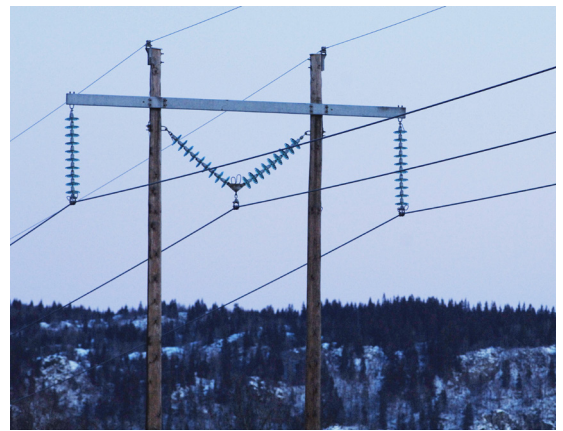
Fig. 5.17: example of an MV overhead line
