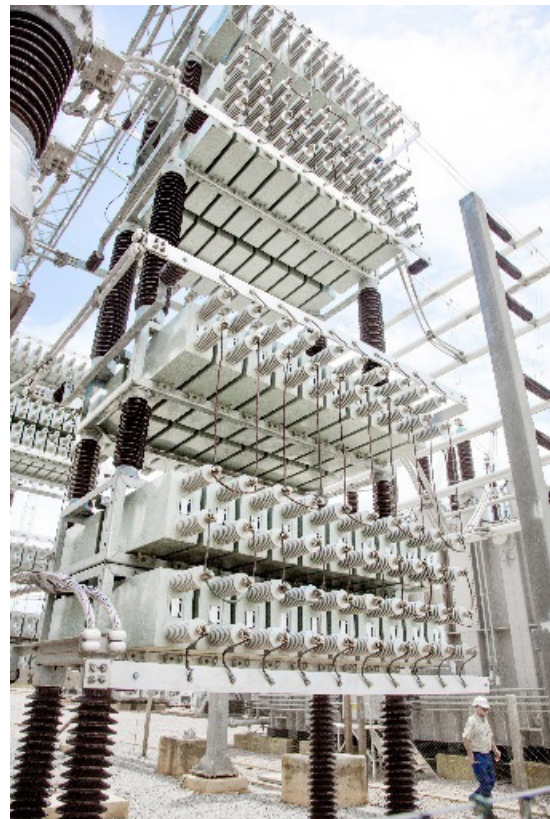
Fig. 5.20: examples of filter banks
