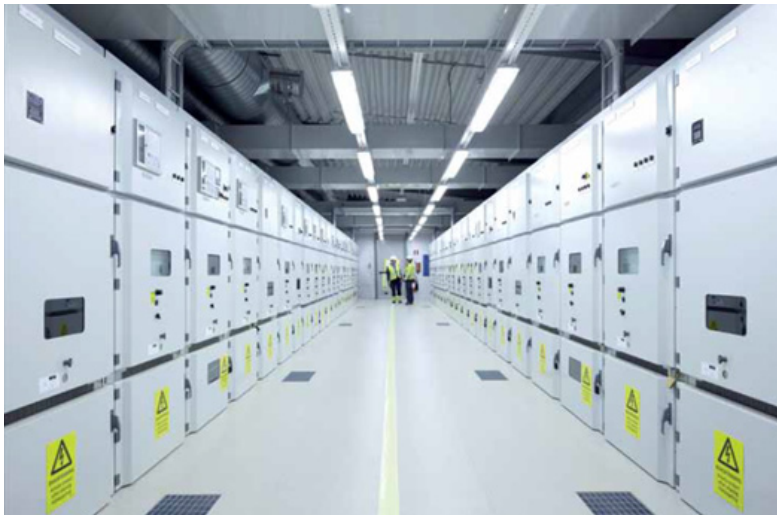
Figure 10: example of an MV substation with UniGear switchgear
