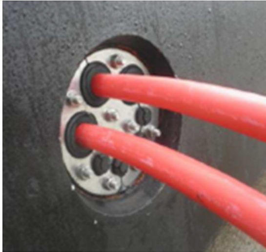
Figure 9: sealed cable entry
