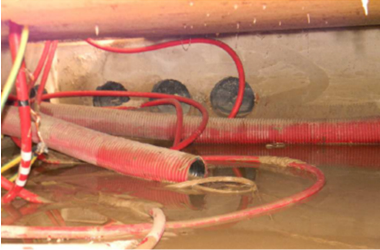
Figure 4: example of a cable cubicle containing water
