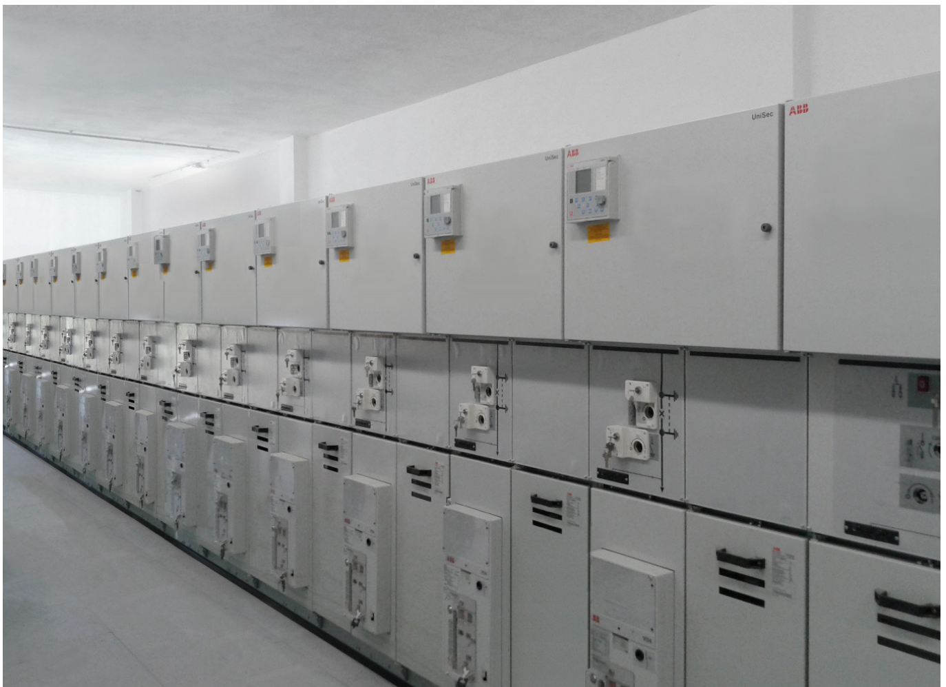
Figure 1: example of a medium voltage substation with UniSec switchgear
