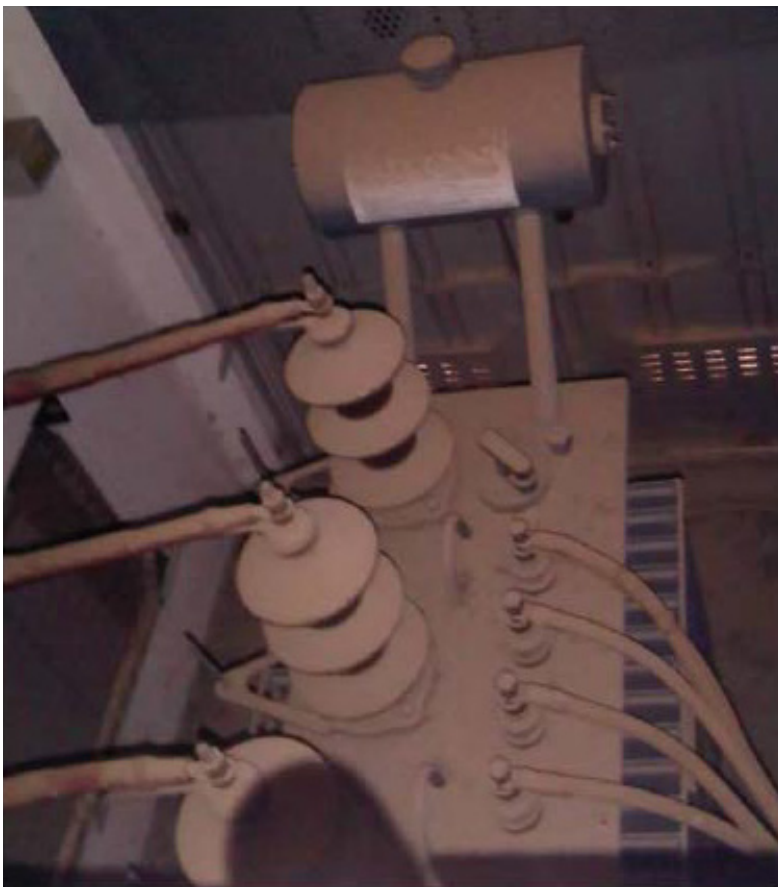
Figure 5: example of a substation where thick dust and other pollutants have built up on the apparatus
