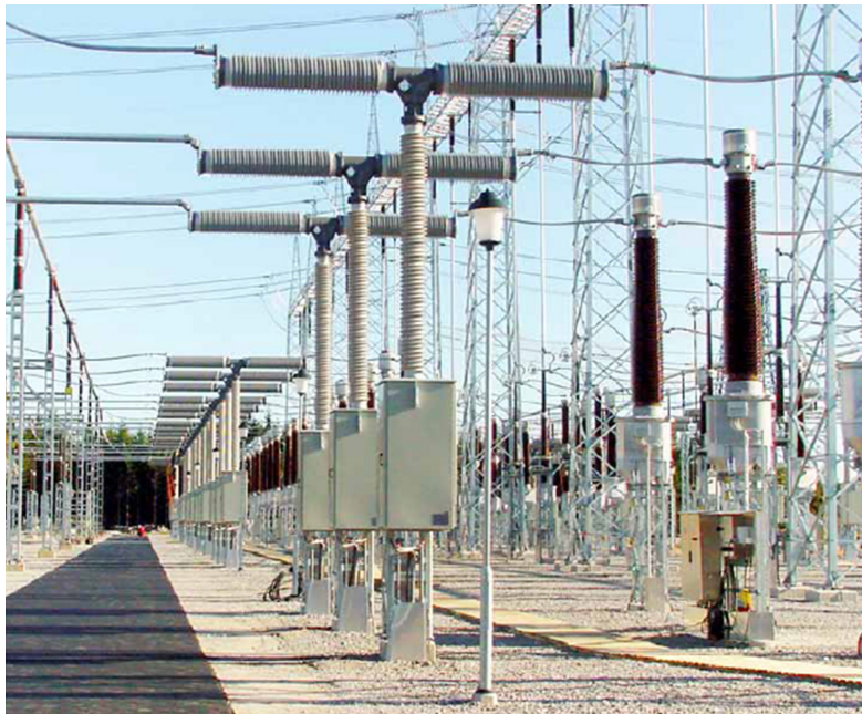
Figure 6: synchronous circuit-breaker in a 420 V substation
