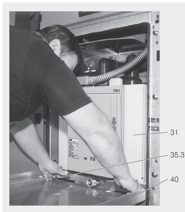
Figure 9/22: Withdrawal of the withdrawable part with circuit breaker onto the service truck.
