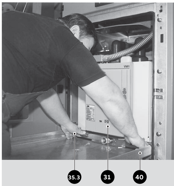
Figure 9/21: Withdrawal of the withdrawable part with circuit breaker onto the service truck.
