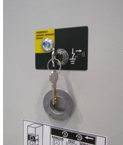
Key lock with key free when earthing switch is open
