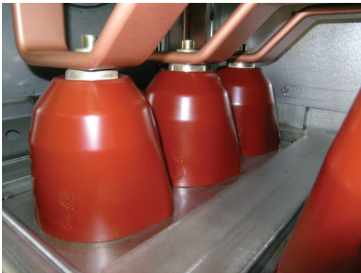
Fig. 7.9.1: View into the circuit-breaker compartment: test sockets
