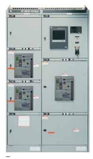
11 AKD-20 LV switchgear with EntelliGuard G breakers
