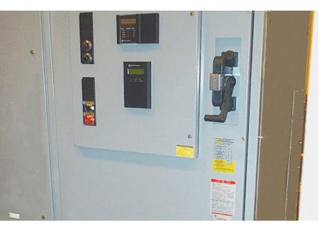
The standard medium voltage soft starter is an SCR-based motor controller designed for the starting, protection and control of AC medium voltage motors. Solid state controllers are available for applications requiring very tightly controlled motor torque and acceleration times and where avoidance of sudden switch-on of inrush current is desired. Reduced voltage soft starter controllers offer several advantages over full voltage non-reversing controllers:
