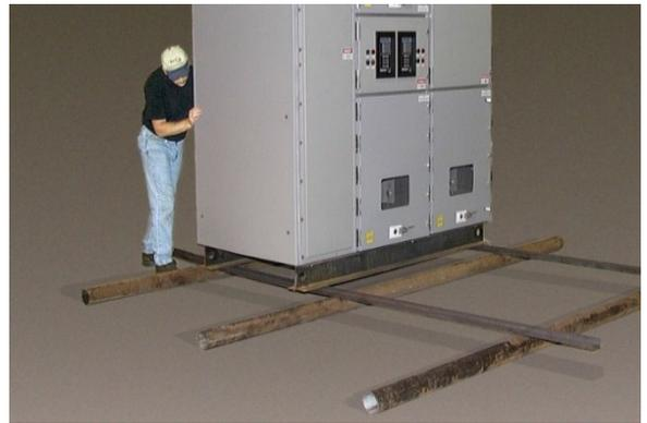
*Figure 9: Lateral movement of the frames with rollers.*
