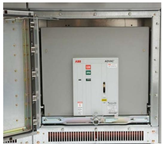
Figure 23: Circuit breaker in DISCONNECT position
