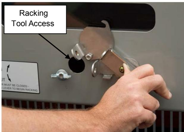
*Figure 24: Racking release handle*
