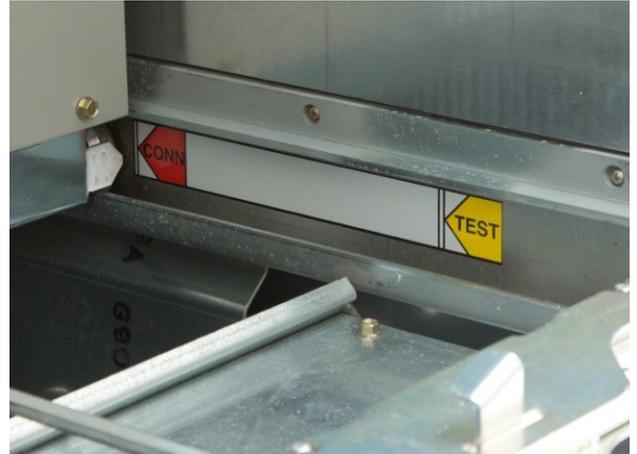
Figure 26:(b) Circuit breaker in CONNECTED position
