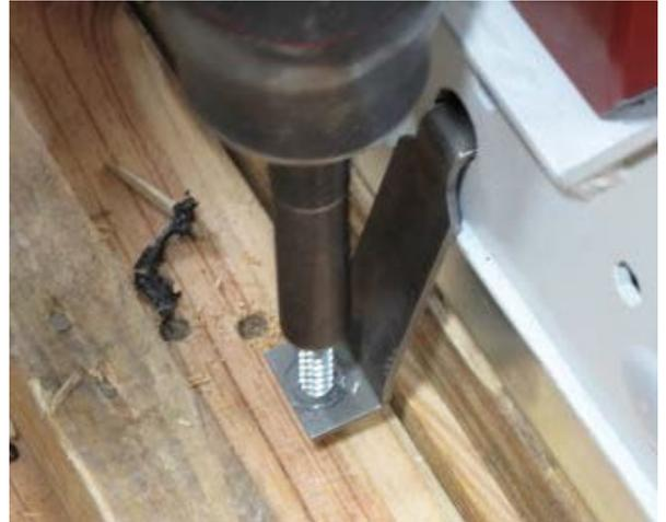
*Figure 15: Clamp screws*
