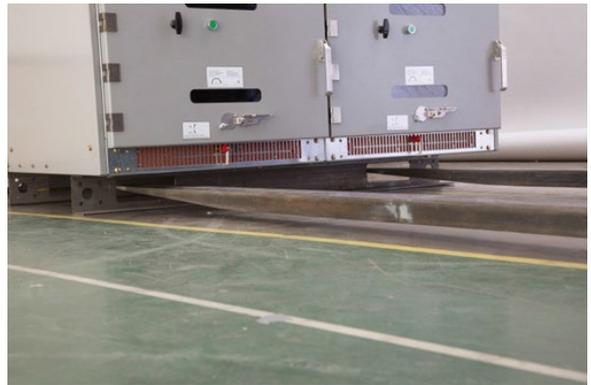
*Figure 3: Forklift forks penetrating shipping channels*
