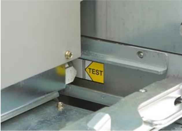
Figure 26:(a): Circuit breaker in TEST position
