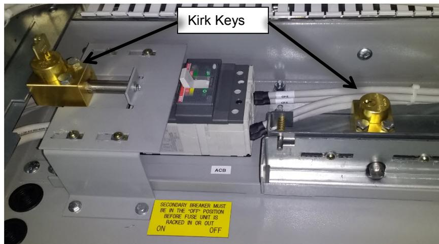
Figure 28: Secondary breaker interlock in 'ON' position and Blocking mechanism withdrawn position.
