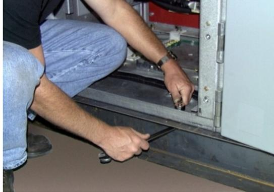
*Figure 10: Unbolting the shipping bases.*
