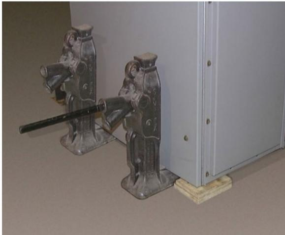
*Figure 11: Using jacks to lower the frames onto wood blocks.*
