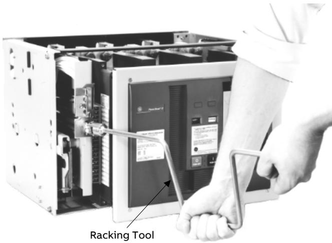
Figure 7. Wrench attached to the device racking shaft.
