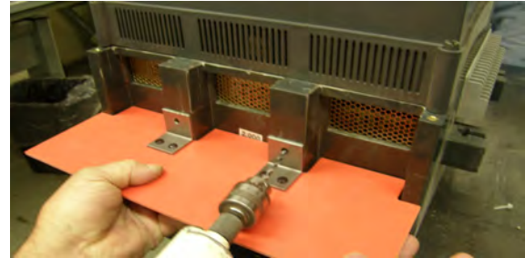
Figure 5: Mark the Area for Drilling Holes
