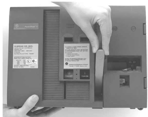
Figure 2: Removing or installing the breaker top cover.
