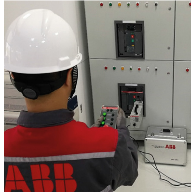
Remote Racking Devices – Emax 2
