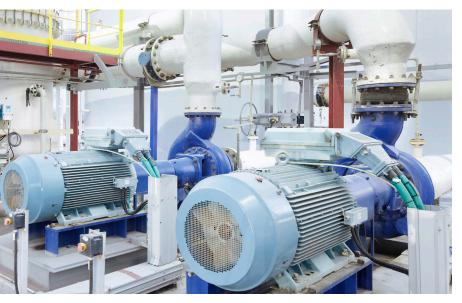
Thanks to ABB's softstartes having torque control, the issue of water hammering when stopping pumps was eliminated. Guhe Electric now saves \$30,000 annually.
