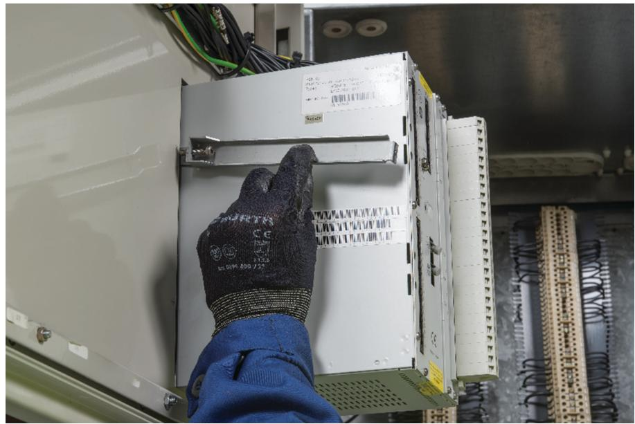
*Figure 5: Detaching the fixing parts of the existing REX 521*
