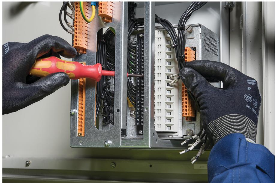
*Figure 32: Connecting the current wires*
