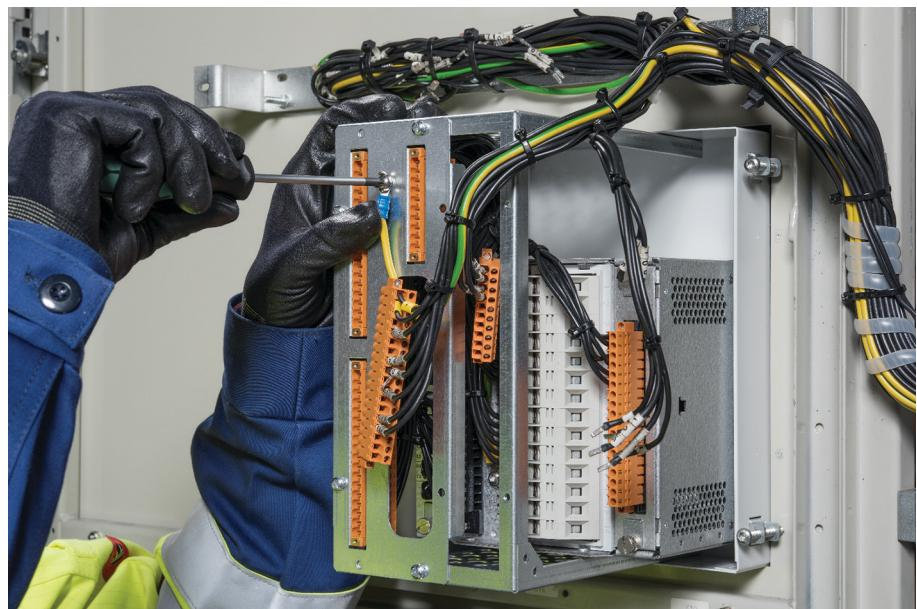
*Figure 28: Tightening the protective earth screw*
