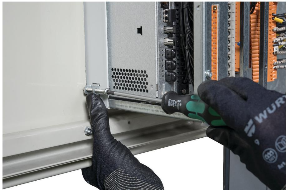
*Figure 16: Tightening the M5 screw*
