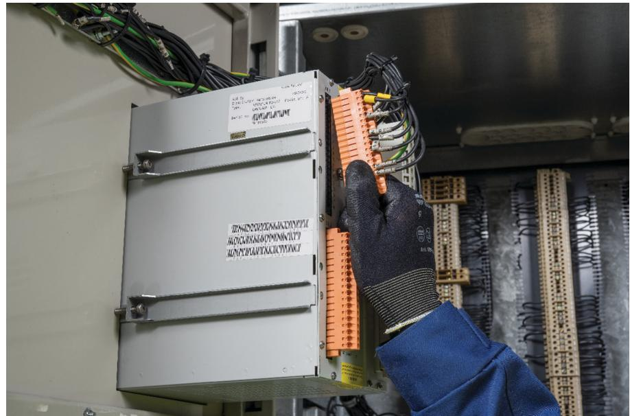
*Figure 2: Removing the existing BIO secondary wiring terminal set*
