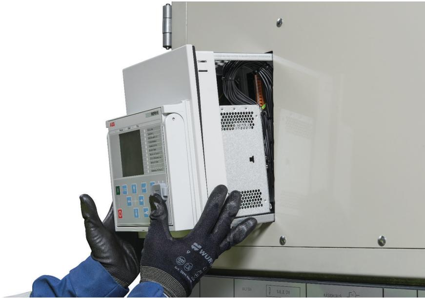
*Figure 11: Mounting REX521RRP into the enlarged panel cutout*
