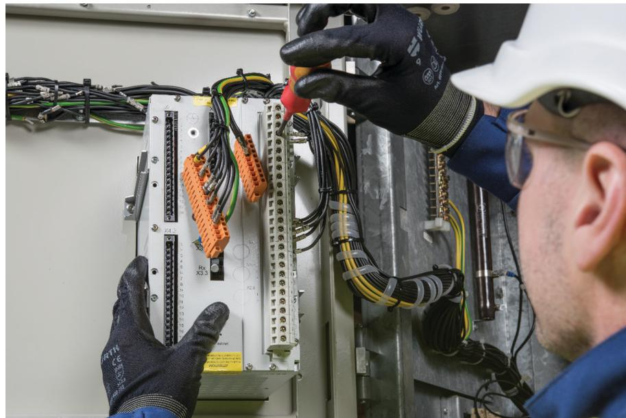
*Figure 3: Removing the existing CT and VT secondary wiring from the REX 521 relay terminal*
