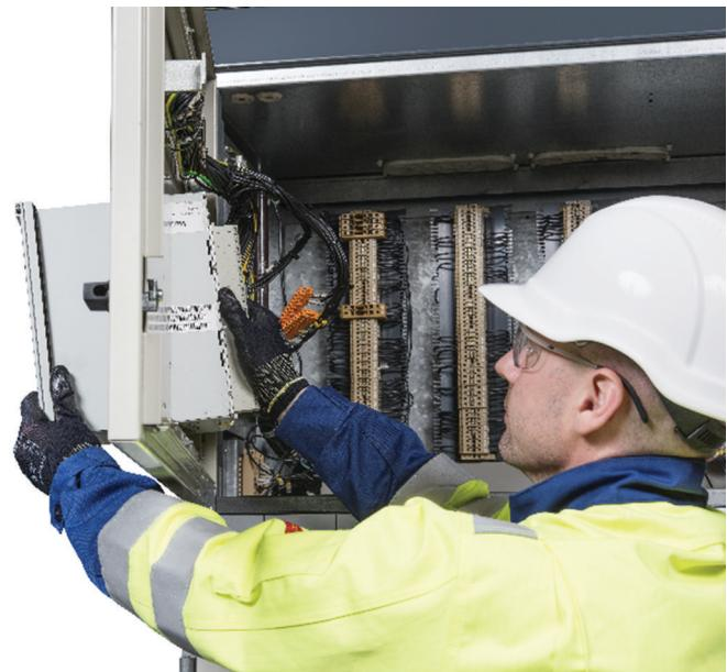
*Figure 6: Taking the existing REX 521 out of the panel cutout*
