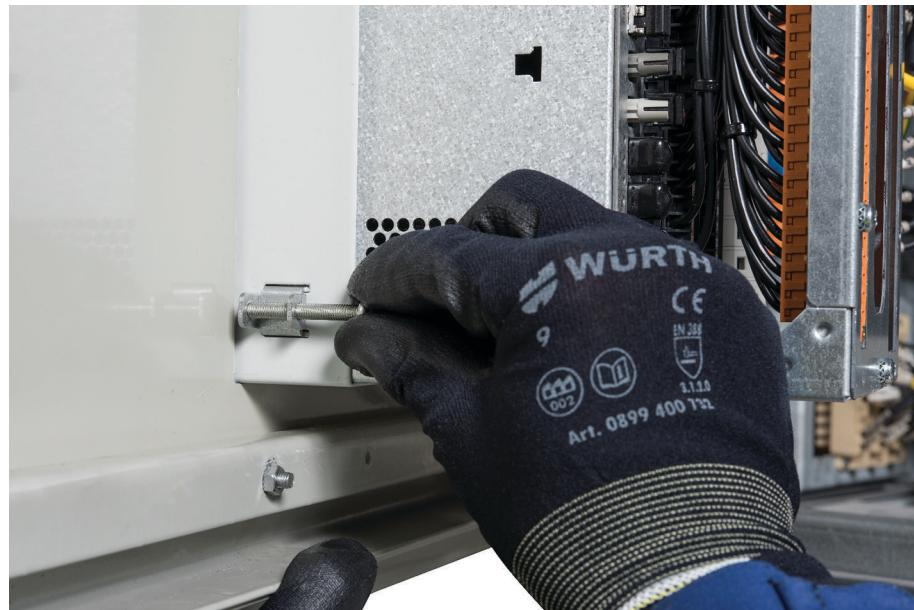
Figure 14: Setting the fixing bracket with the M5 screw
