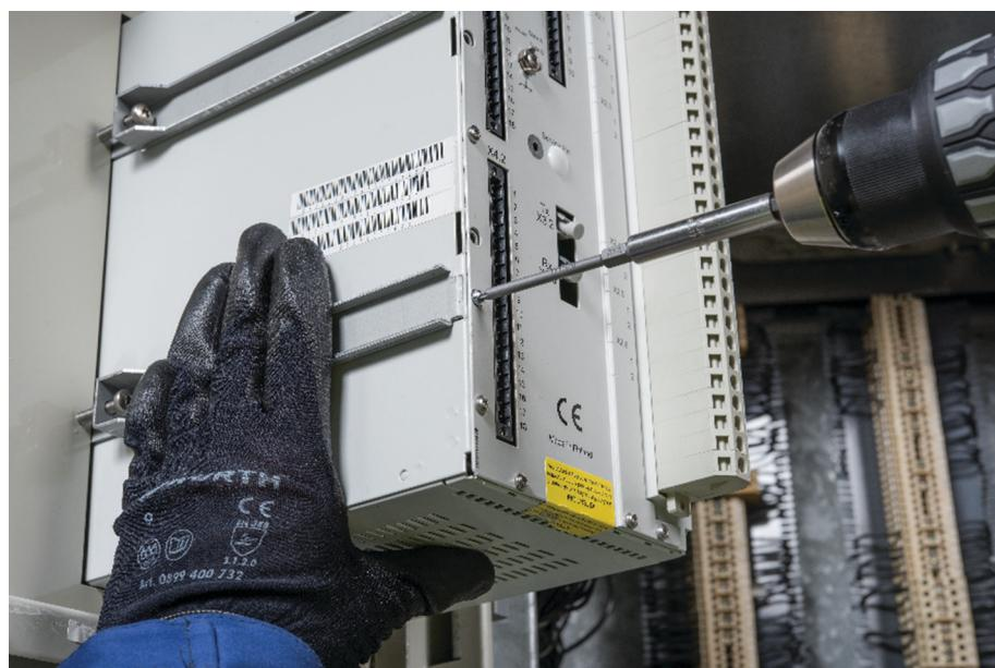
*Figure 4: Taking the existing REX521 out by using the appropriate tools*
