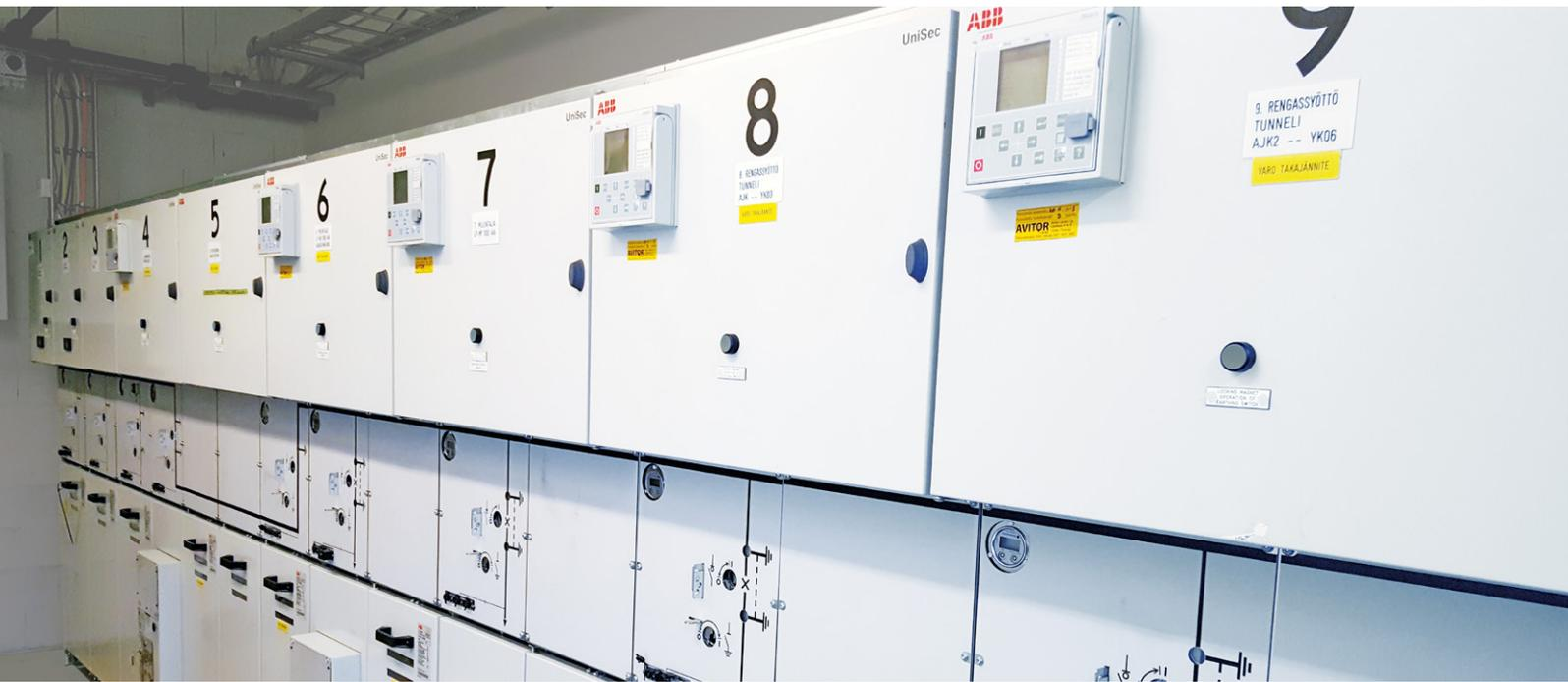
If there is a complete power outage from the external power supply, the protection relays give a start command to activate the reserve power system. The restoration of the power distribution grid in the tunnel is then done automatically in the MicroSCADA Pro system.
