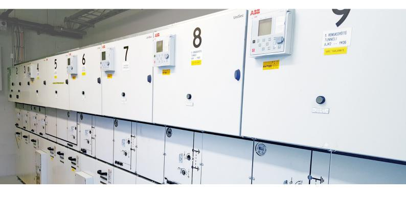
If there is a complete power outage from the external power supply, the protection relays give a start command to activate the reserve power system. The restoration of the power distribution grid in the tunnel is then done automatically in the MicroSCADA Pro system.
