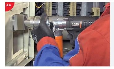
Cut the parts next to the edges first and the middle part last.
