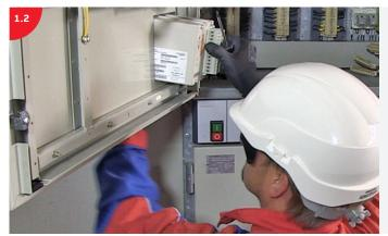
Start by removing the existing relay.
