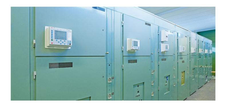
The 630 series IEDs and REA arc protection system were installed in the MEKA 24 switchgear.
