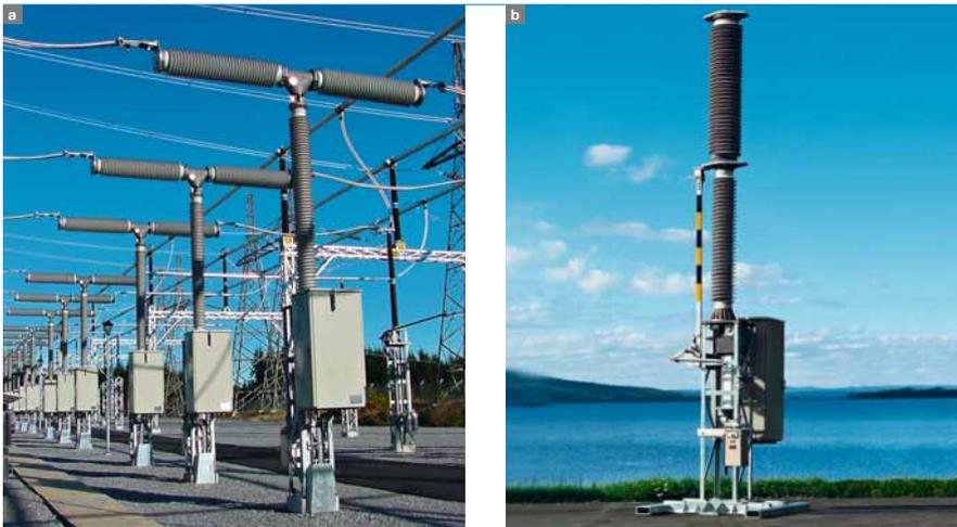
5 Space requirement of 145 kV substation (traditional) a compared to the same functionality achieved with the “Combined” breaker b
