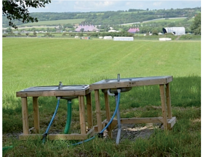
1 The Glastonbury Festival draws more than 177,000 people a day. Photo: Andrew Allcock. | 2 A network of pipes distributes water from underground reservoirs to hundreds of hand basins and taps around the site.
