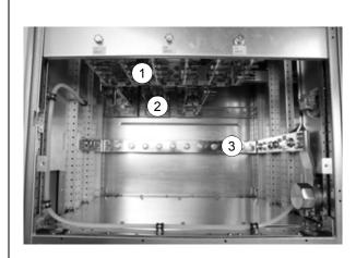
Cable connection terminals and cable entry plate (blank plate)
