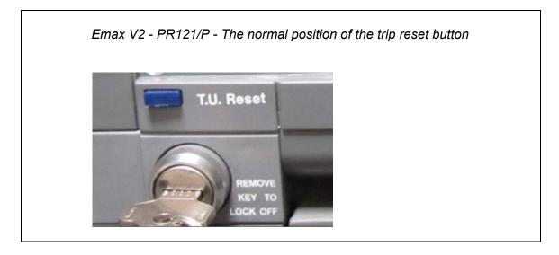
When MCB TRIP appears for the first time, there is a speed warning following MCB TRIP fault in the fault logger of the rotor-side converter. If the PLC continues making automatic reset trials after MCB TRIP and TU-TRIP button is out, the fault logger will fill up with MCB TRIP indications and speed warning is not shown anymore.
