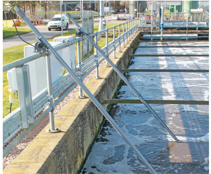
Both standards use a scattering angle of  $90^\circ$ , which is called nephelometric arrangement, but each of them use a different wavelength and different prescriptions on the geometry of the illumination and detection. Using detection at  $90^\circ$  reduces the effect of stray light and absorption.
