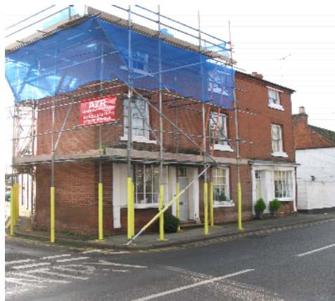
Vertical uprights and bracing
