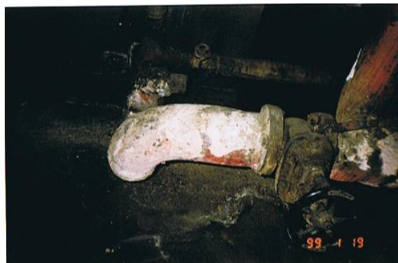
Damaged asbestos thermal insulation on pipework
