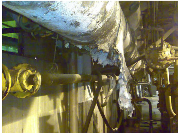
Damaged asbestos thermal insulation
