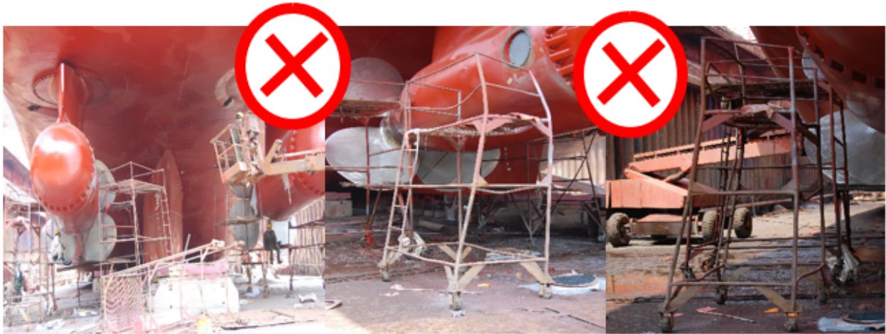
Figure 16.2: Damaged and dangerous mobile scaffolding
