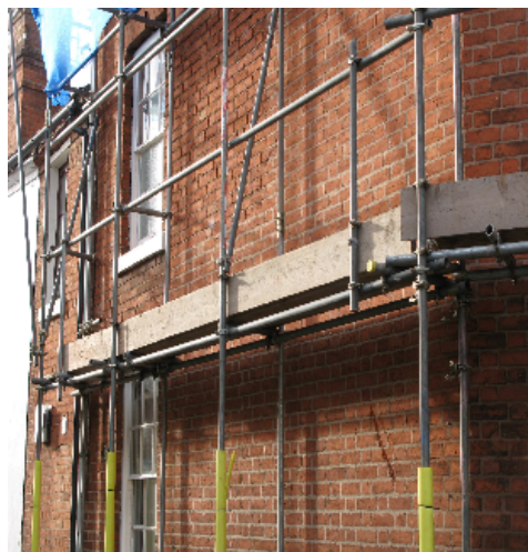
Platform, toe board, rails
