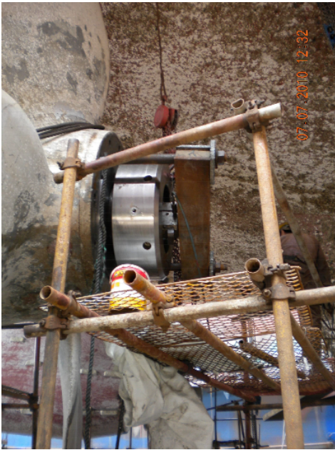
Fixed scaffolding in dangerous state
