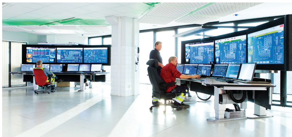
The ABB 800xA distributed control system technology enables collaboration and remote operations in a central location. (Photos courtesy of ABB)
