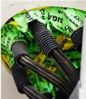
Up to 15 DC power cables are therefore well protected inside the conduit and guided into the building. With this in mind, it was quite clear for René Künzli, head of photovoltaic solutions at BE Netz AG, that the PMA conduits from ABB had to be used once again for this extraordinary project.
