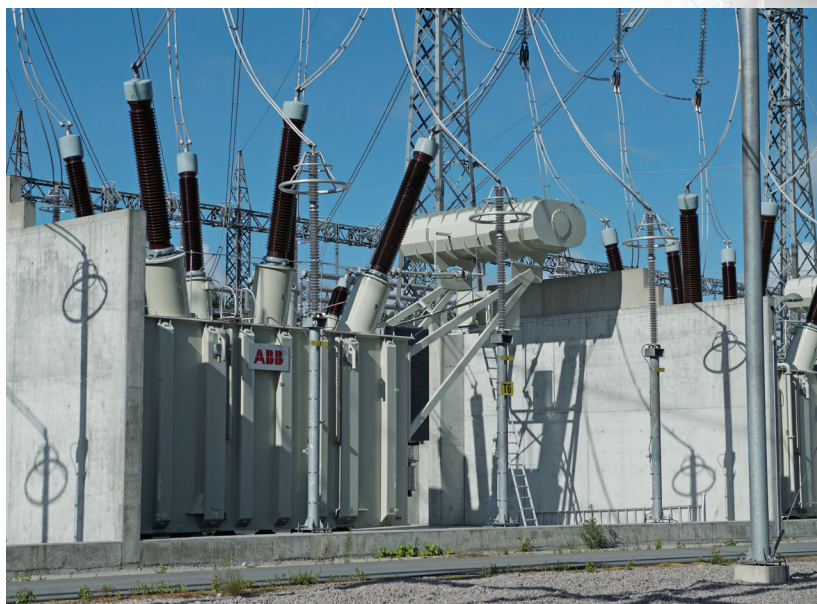
Figure 7: This large power transformer could be impacted by GMDs produced from solar flares.
