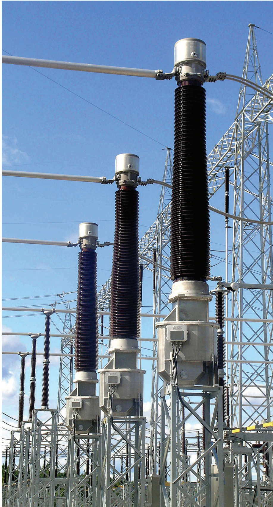
420kV Oil-Filled Current Transformers
