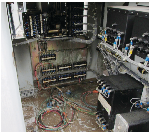
03 A water-logged control cabinet is pictured here.
