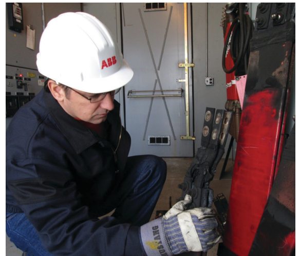
02 The switch gear had not been disengaged, and equipment was damaged.
