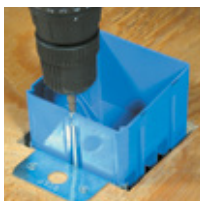
2 Screw in to adjust to height of flooring or carpet.
