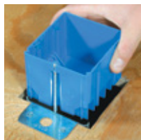
1 Install clip over subfloor.
