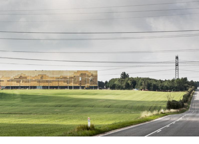
01 Skagerrak 500 kV HVDC Light Hybrid bipole, converter building.
