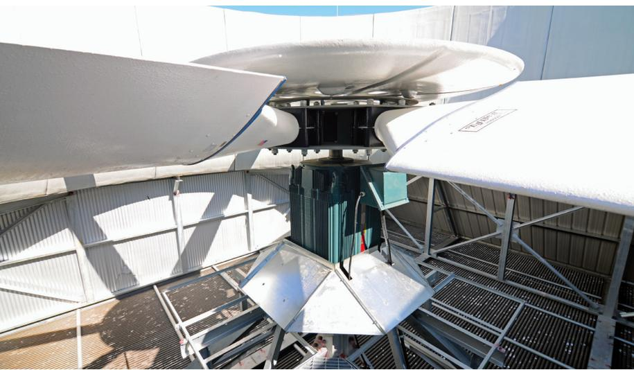
Cooling towers are used in food processing plants all over the world. Maintenance and failure of the gearbox, and associated components, is often problematic with traditional systems. The Baldor-Reliance® RPM AC direct drive cooling tower eliminates these problems by coupling the motor directly to the fan and controlling it with a unique drive.
