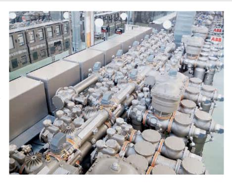
The fluoroketone-based gas mixture for switchgear applications was developed in collaboration with 3M. This fluorinated molecule decomposes under ultraviolet light in the lower atmosphere, giving a lifetime of around 15 days, versus 3,200 years for SF<sub>6</sub>. The global warming potential (GWP) of the gas mixture is below 1. In a joint pilot project with ewz, a leading Swiss utility, the world's first
