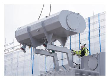
From the installation of an ABB transformer at the new converter station at Kollsnes in Hordaland.
